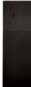
Panel Skirt Completely Installed
