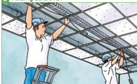
2 Installing Canalis KDP
