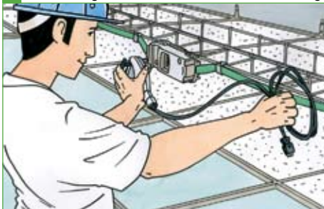
4 Connecting the connector to the busbar trunking
