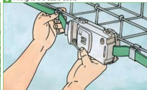
3 Fixing to the cable ducts
