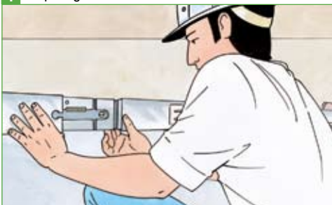
1 Preparing a set of busducts on the floor
