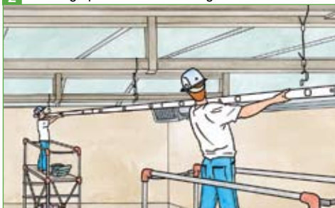
2 Hooking up the busbar trunking
