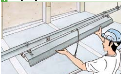
4 Fitting the lights
