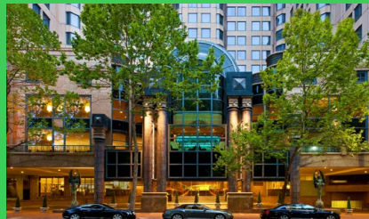
Sheraton on the Park saves 15% on energy bill thanks to EcoStruxure™ Building upgrade
