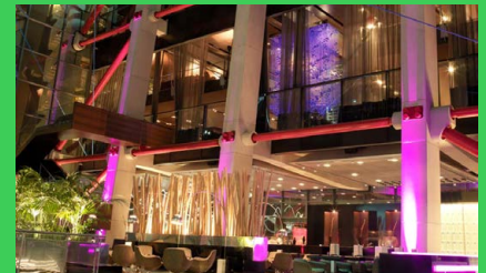
Barcelona Tower Hotel achieves 30% energy savings with EcoStruxure™
