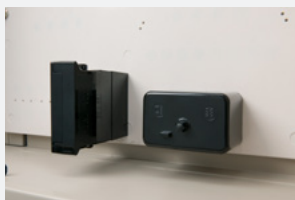
Service fuse holder and neutral link
