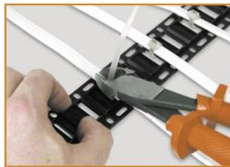
**4** Cut off the excess from the cable tie.
