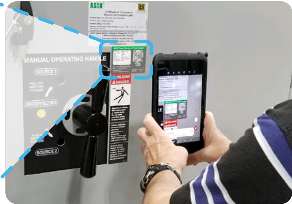
Any QR code reader can be used to access basic serial number-linked information about a transfer switch.
