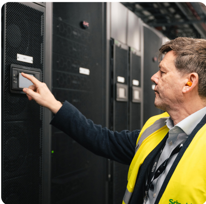
Schneider Electric APC InRow Cooling
