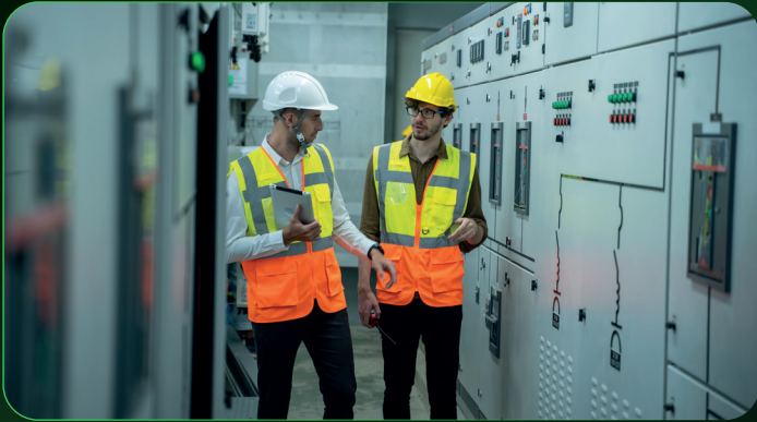
Distribution and Power Generation
