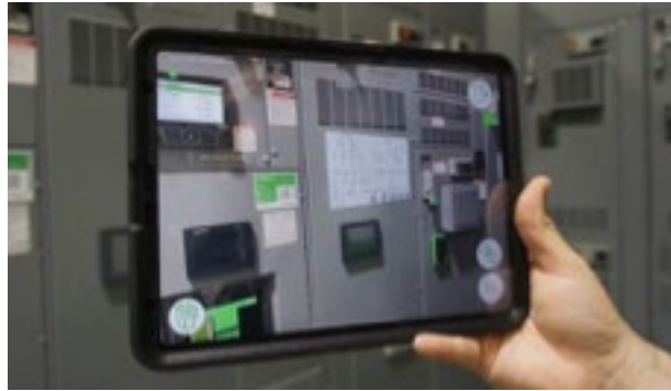
Figure 20. An AR system can quickly find and reveal other required documentation or information, such as a virtual schematic that can be correlated with switchgear operation
