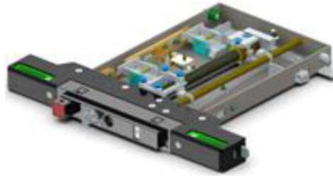
The purpose of this truck is to enhance reliability by integrating a new rack-in system of medium voltage circuit breaker in an existing AIS cubicle. Some particular points of this study were:
