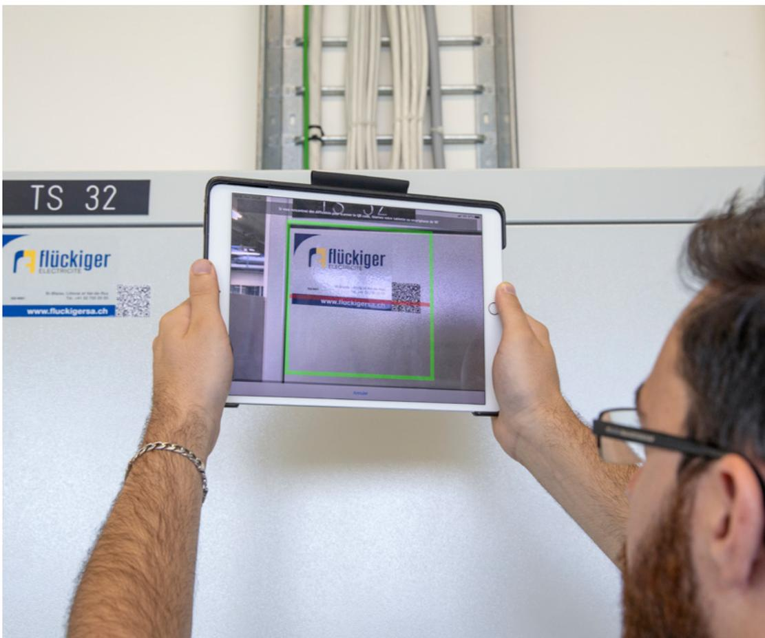
“By scanning QR codes, the technical team saves time on locating the equipment to be maintained and can quickly access its digital maintenance log.”
