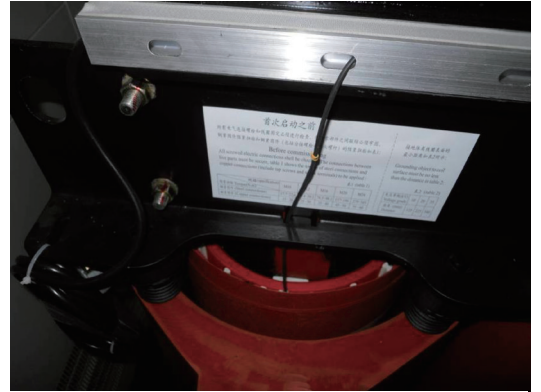
Figure 16.1.1: Sensor (PT100&PTC150)
