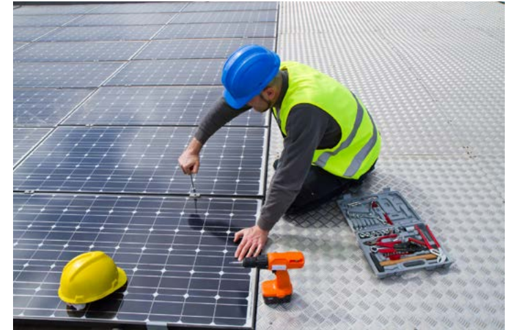
Setting and enacting a sustainability strategy is easier with the right data. In fact, many tenants are making it a point to choose locations with green buildings initiatives.
