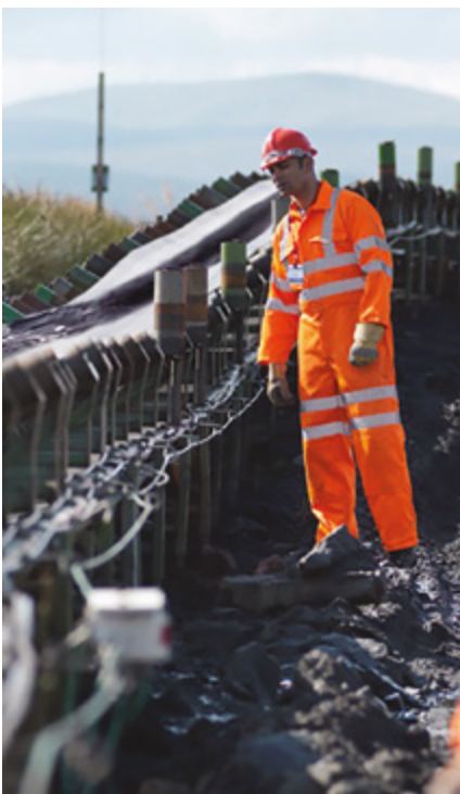
3-level AFE for long belt conveyor application
