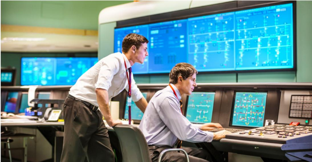
An ADMS deployment provides operators for Austin Energy with a real-time view of system data, crew locations, and SCADA and OMS information.
