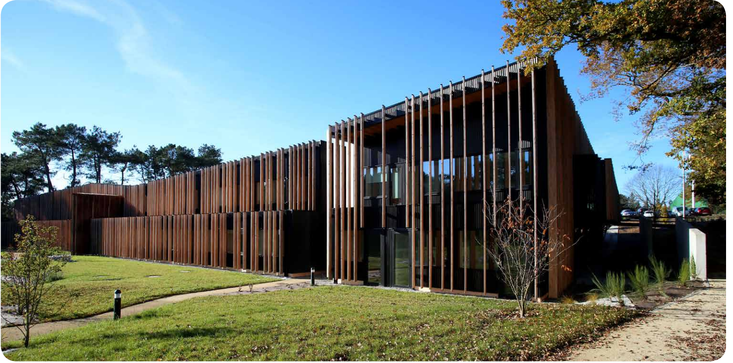
The modern SDEM headquarters in Vannes, France, features over 800 m 2 of roof-mounted solar panels, plus two small wind turbines.
