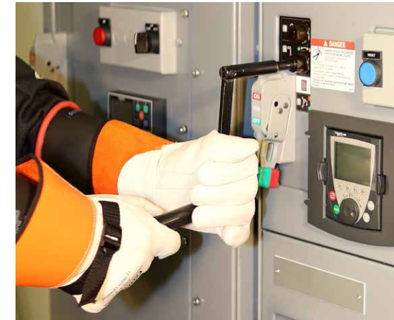
Racking handle (same as Masterpact™ NT/NW breakers)
