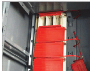
Figure 7: Removing the Manual Bus Shutter
