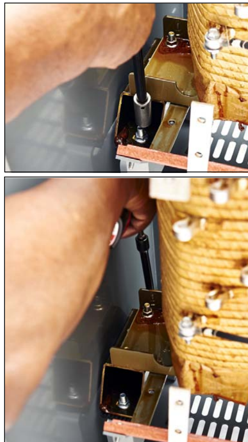
Figure 27: Enclosure Style K: Bolts Accessible from the Front of the Transformer
