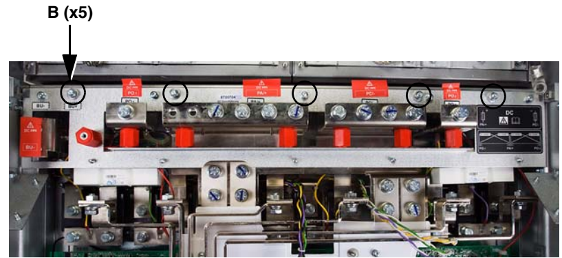
Figure 72: Bus Bar Connections
