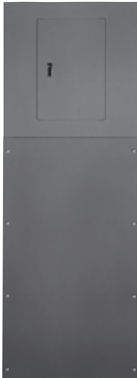
Panel skirt completely installed.
