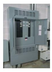
• 15 KVA 480/208 V Transformer: A wall mounted transformer to create 208.120 Volt supply for house loads such as lighting, fire suppression, and convenience outlets
