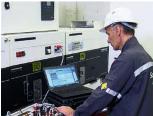
OnSite ProDiag MV Relay diagnose the condition of the electronics and configuration settings on medium voltage protection relay
