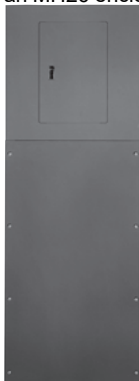
Panel skirt completely installed.
