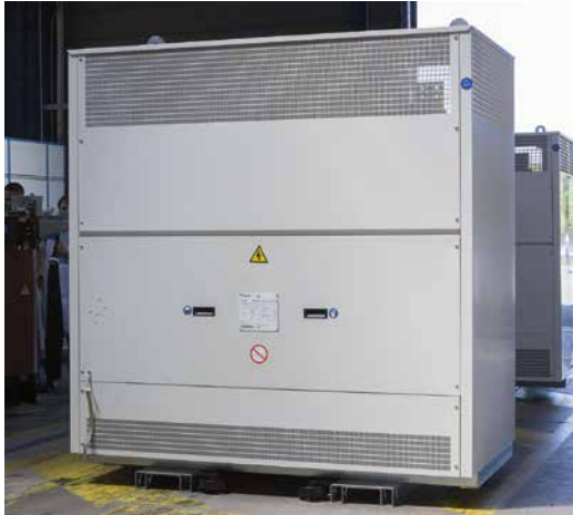
Protective enclosure IP31, IK7
