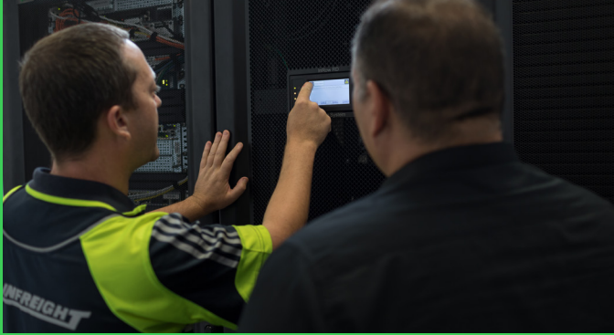
EcoStruxure for Data Center
