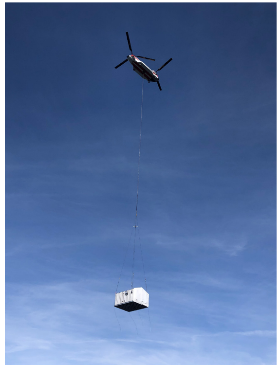
Transportation of equipment storage shed via helicopter to remote mountain-top telecommunication site.
