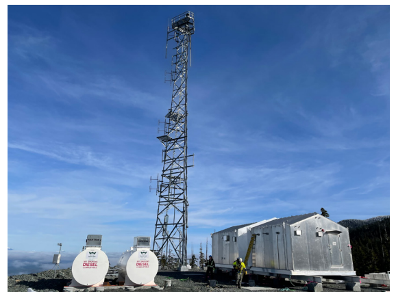
Final site assembly: mounted communication tower, power and communication equipment storage, and diesel storage tanks for generator fuel.
