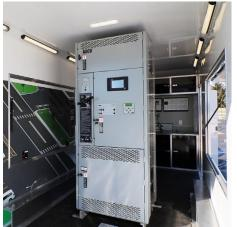
The trailer is equipped with an ASCO 600-amp 7000 Series H-Frame Isolation Bypass Transfer Switch. View its design; operate, bypass, and isolate the transfer switch; and evaluate the working controller and Touch Display Interface.
