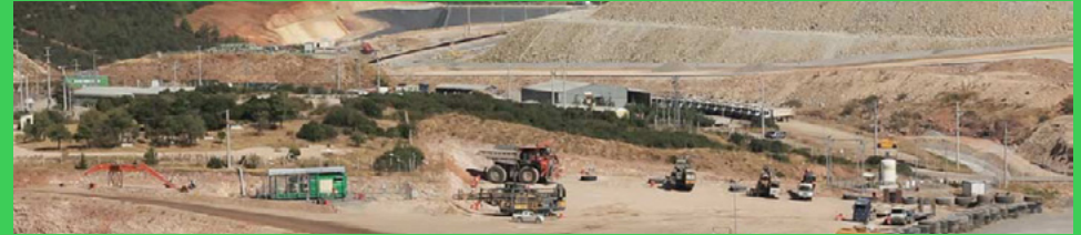
Tuprag Mine ensures reliable power
