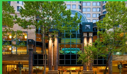
Sheraton on the Park saves 15% on energy bill thanks to EcoStruxure™ Building upgrade
