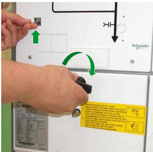
Lift the pull control device to unlock the panel. Pull out the panel to the right.
