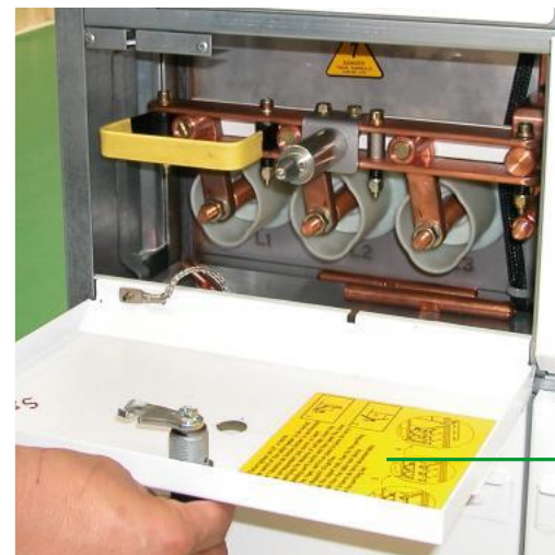
Pull the panel forwards to remove. Note: A second instructions label (3) describes the rest of the operation.
