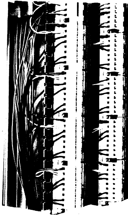
Figure II-11. Field Wiring in I/O Housing Conduit
