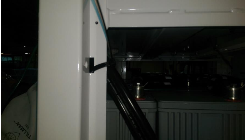
Figure 39 : Intershelf cable tied to frame
