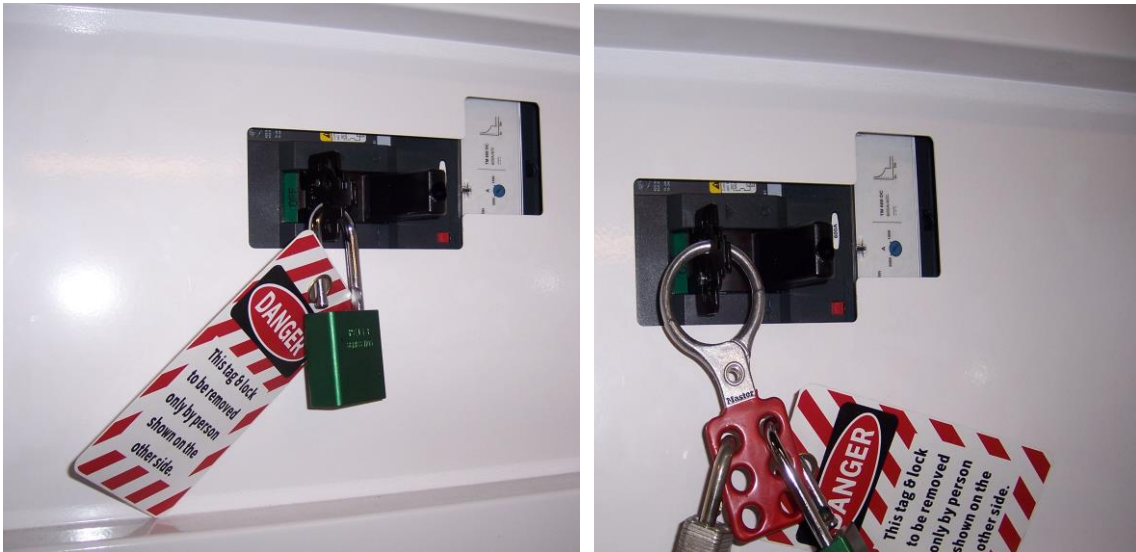
Figure 48 : Lockout attachment installation
