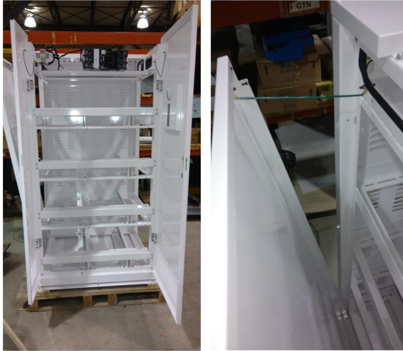
Figure 41 : Reattachment of the green ground wires
