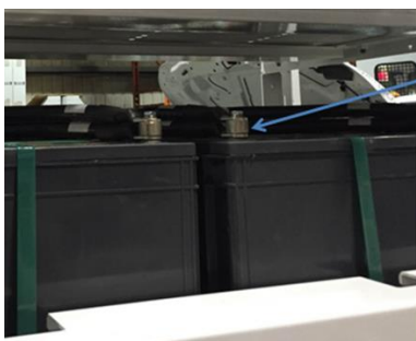
Double run configuration with copper spacer
