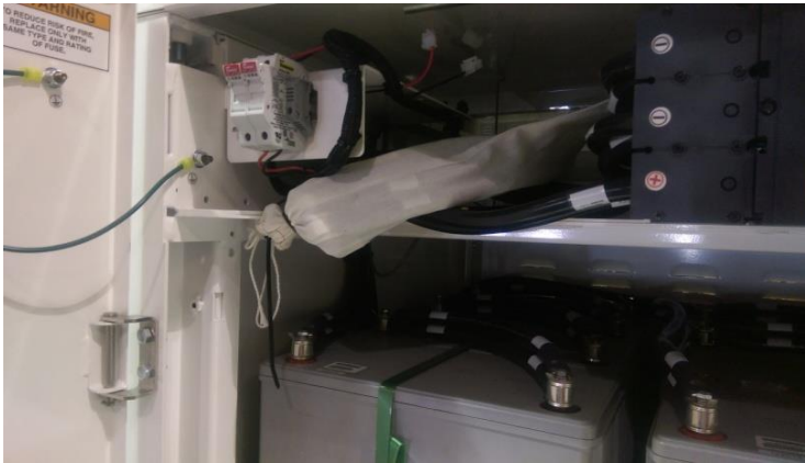
Figure 42 : Bagged cables placement
