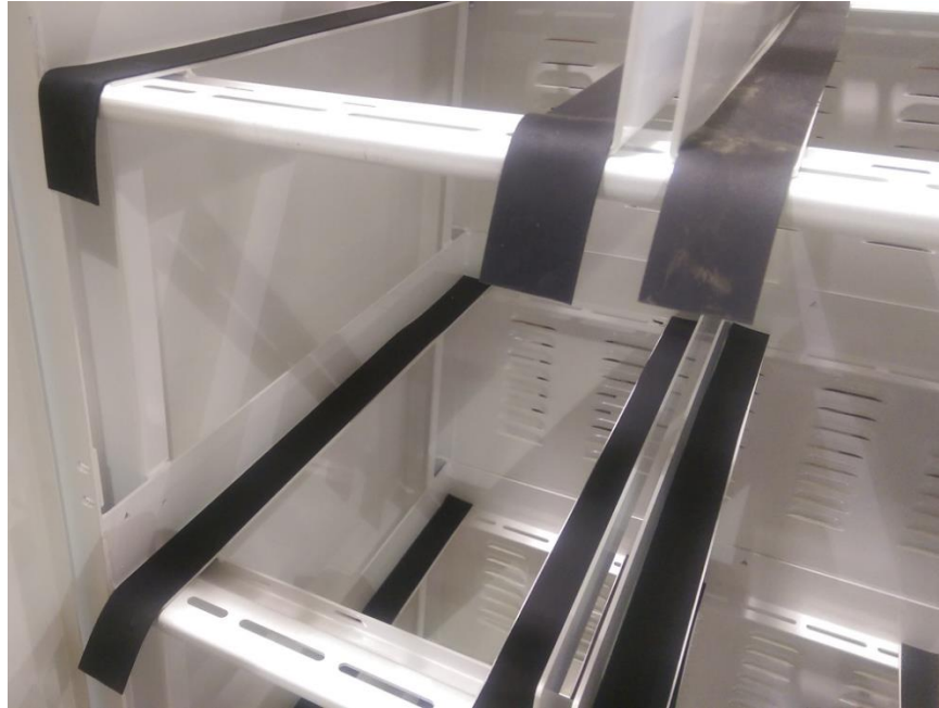
Figure 5 : Placement of Santoprene strip
