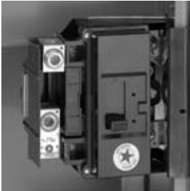
QOM2200MVH Bolt-On Circuit Breaker Installed
