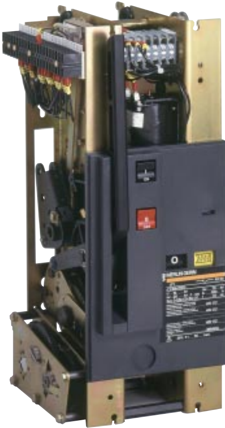
RI operating mechanism.
