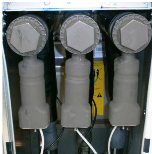
Figure 6. Typical GIS architecture including LPVTs
