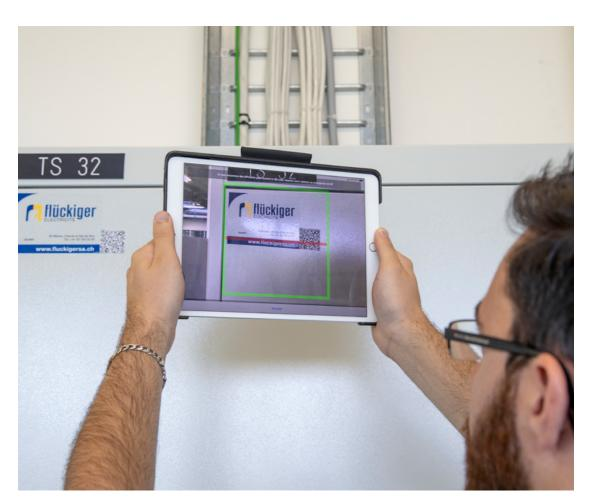
"By scanning QR codes, the technical team saves time on locating the equipment to be maintained and can quickly access its digital maintenance log."
